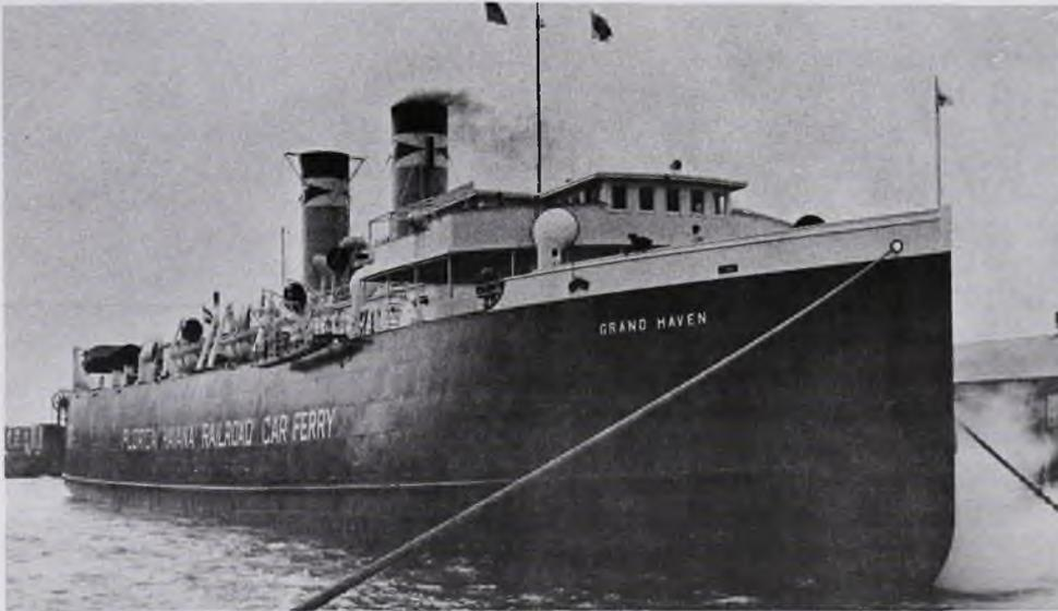
**Above:** GRAND HAVEN (US 200007, Hond. 2180). Built: 1903 by Craig S.B. Co. (#92), Toledo. Measurements: 2320 gt, 1678 nt; 307 x 54 x 20. Engines: 2 triple-exp., 22"-36"-61" x 36". Boilers: Originally 8 scotch, 11½ x 11½; replaced 1952 with 4 B & W water tube boilers built 1919-20. Owners: (1) Crosby Car Ferry Co.; (2) Grand Trunk Milwaukee Car Ferry Co.; (3) West India Fruit and Steamship Company, Inc. —Massman photo
