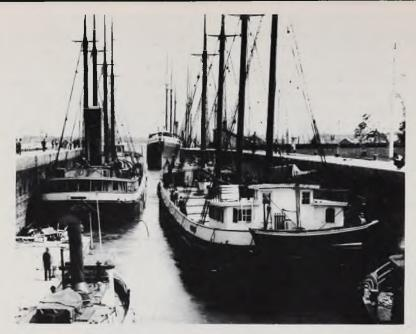
Iron Duke was powered by a Frontier Iron Works Steeple Compound engine with 26" and 48" cylinders and 36" stroke. She was fitted with "an American ship windlass worked by steam, the first of the kind on the lakes." At right is the schooner barge Iron Cliff, also of 1881.
