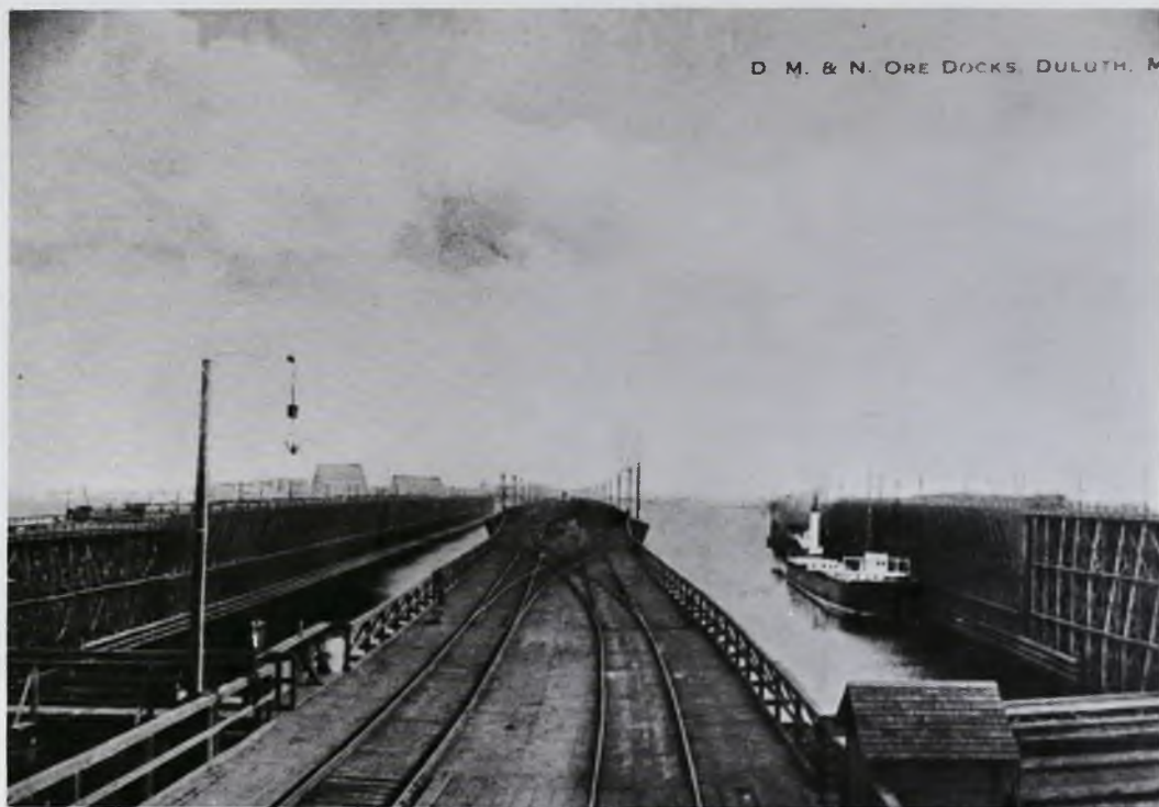
'The longest ore docks in the world,' about 1902. The freighter at right is the 430-foot MAUNALOA.
