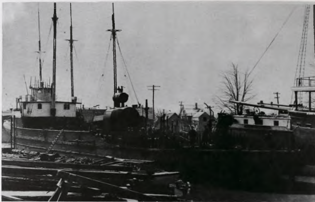
SAKIE SHEPARD at Marine City for repairs after fire.
