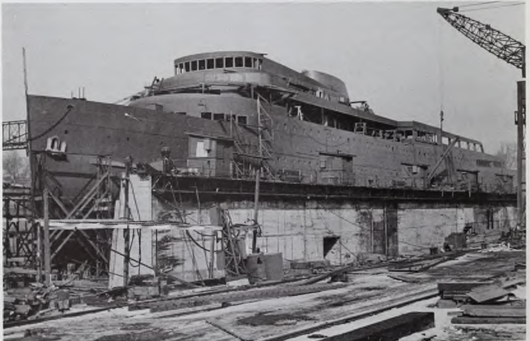
JUNIATA at Manitowoc, April, 1941, with new superstructure well on the way to completion.
