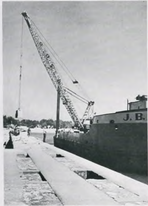
J.B.II engaged in rehabilitation work on South Breakwater, Muskegon, Michigan, in 1968.
