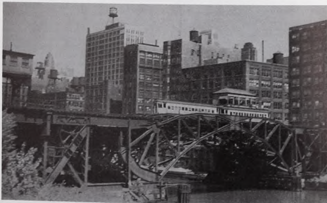
Fox Valley Limited. . . Chicago, Aurora & Elgin interurban train stamps across elevated railway bridge moving toward far west suburbs. Now removed, this Scherzer-type bridge was almost unique. One word for the interurban — FAST!
