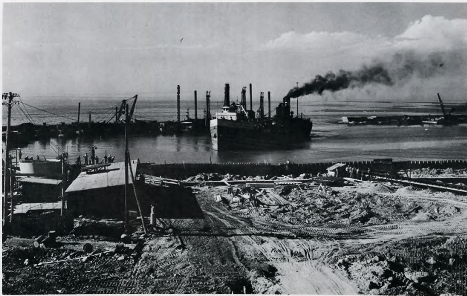
The JOSEPH S. SCOBELL arrives in Oswego with the first boatload of coal from Sodus Point on July 9, 1940. Work on the dock had not yet been completed, and coal was unloaded onto a temporary conveyor belt.
