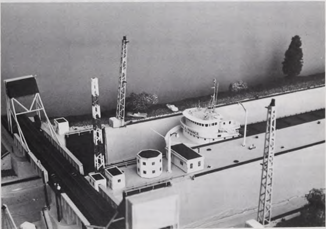
Close up view of the railroad bridge at Lock 4.
