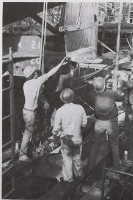
Left: Workmen stand over shaft as a crane lowers the new blade. Right: Welder repairs damaged frames in the port side.
