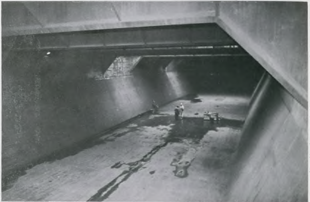
Work completed in number two cargo hold, which measures twelve feet shorter than a football field.
