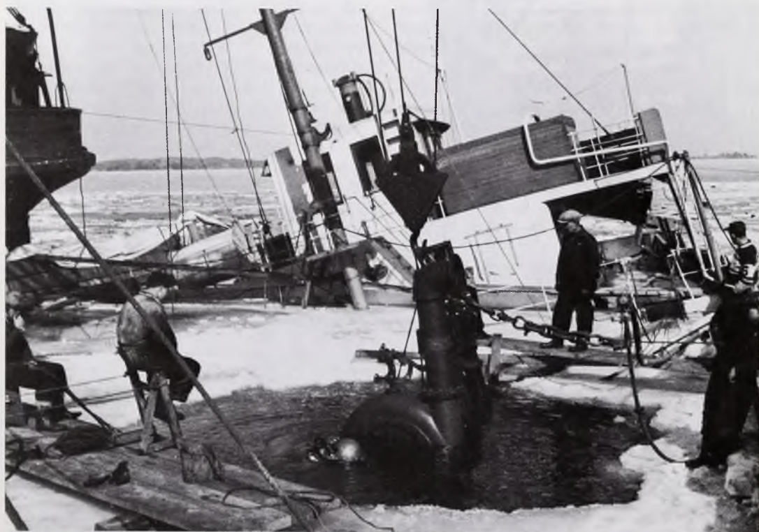
Pump is lowered into the cargo hold on March 12.
