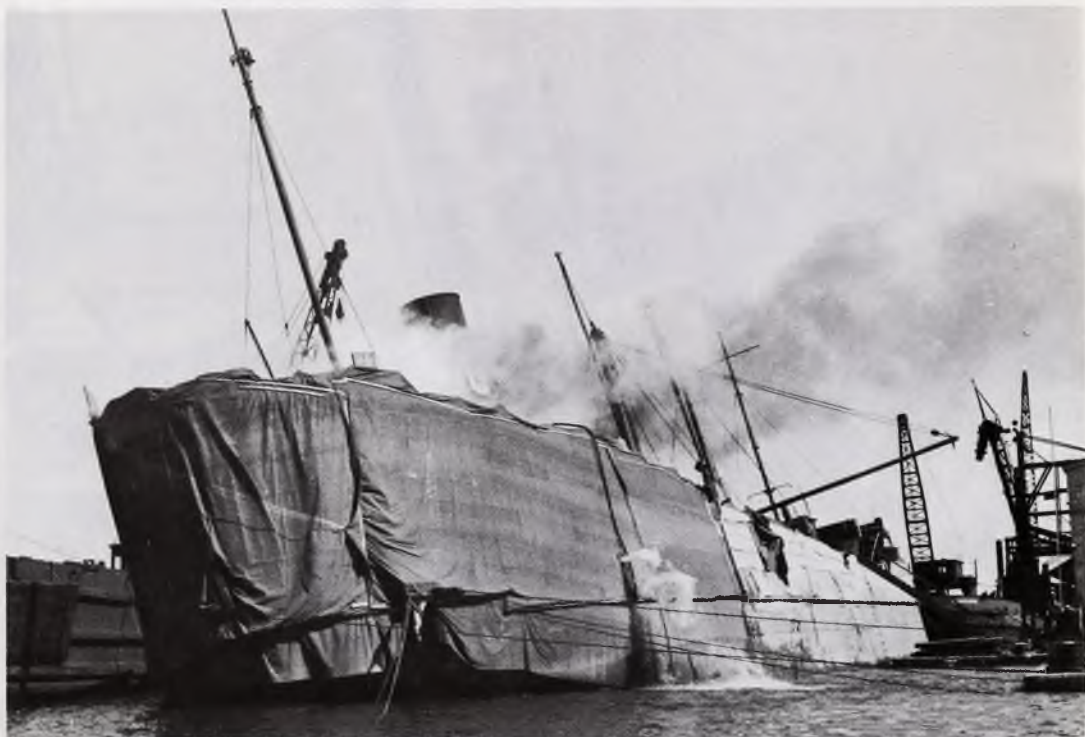
Lines are secured tightly as the OUTARDE is pumped out on April 19.
