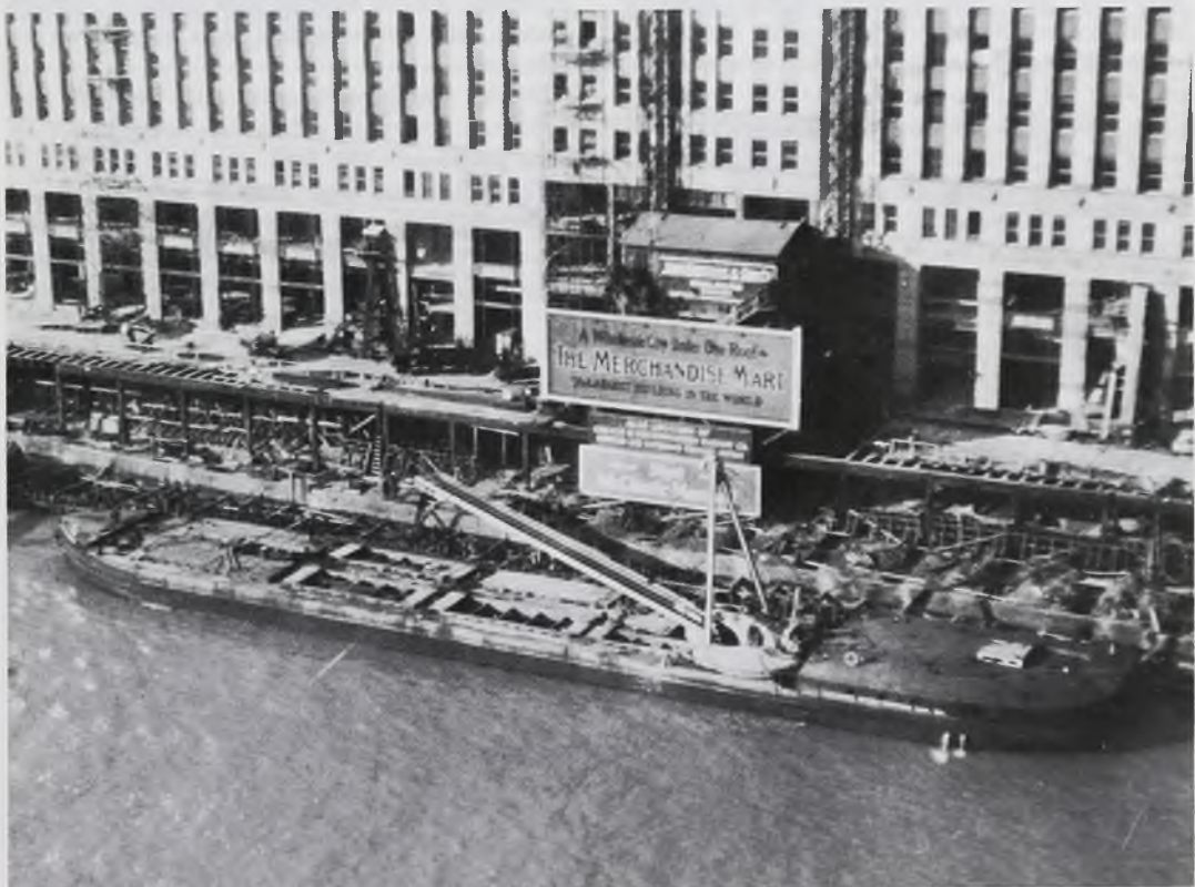
MATERIAL SERVICE fills in the riverfront caissons at the construction of the Merchandise Mart in 1931.
