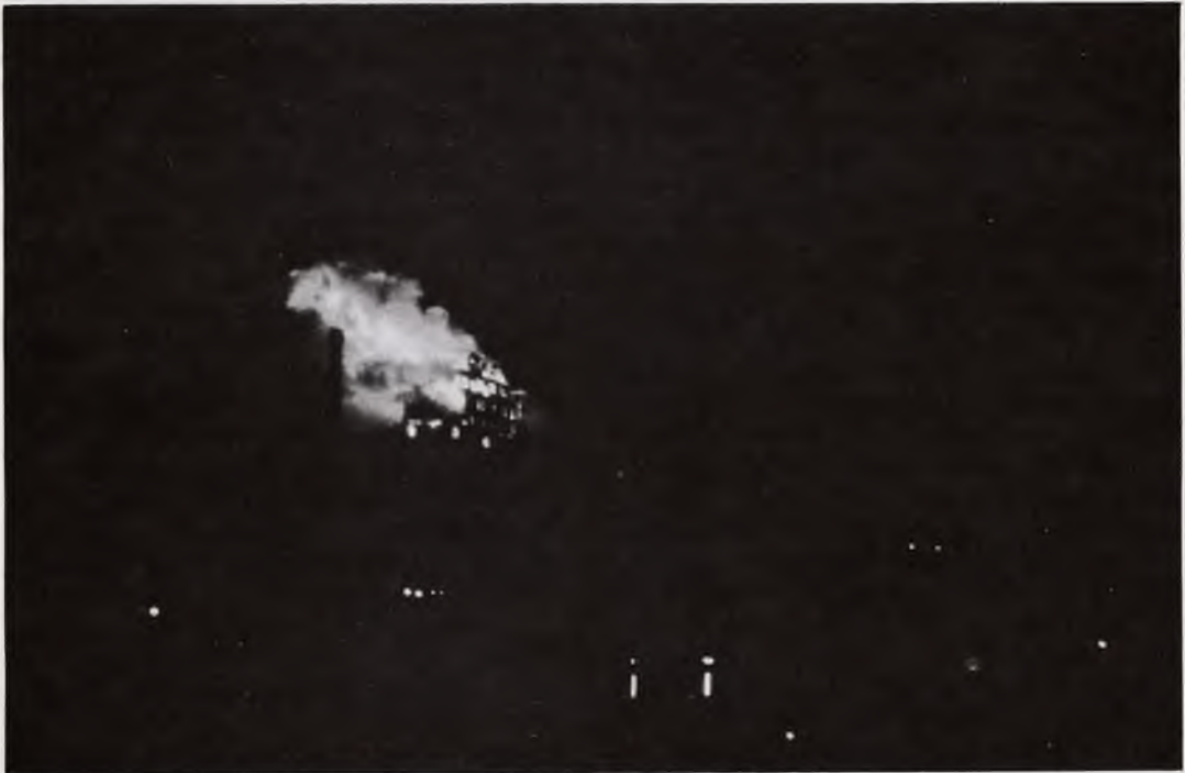
Continental "A" Elevator burning fiercely in January, 1957. Blazing frame structure created enough light that one could read a newspaper by it a half mile away.
