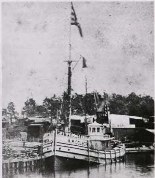
*A.R. COLBORN* was built in 1882 with a 240 horsepower steam engine. Note the pilot house on stern.
