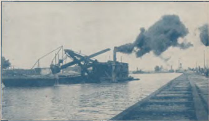
Dredge at Work in Channel
