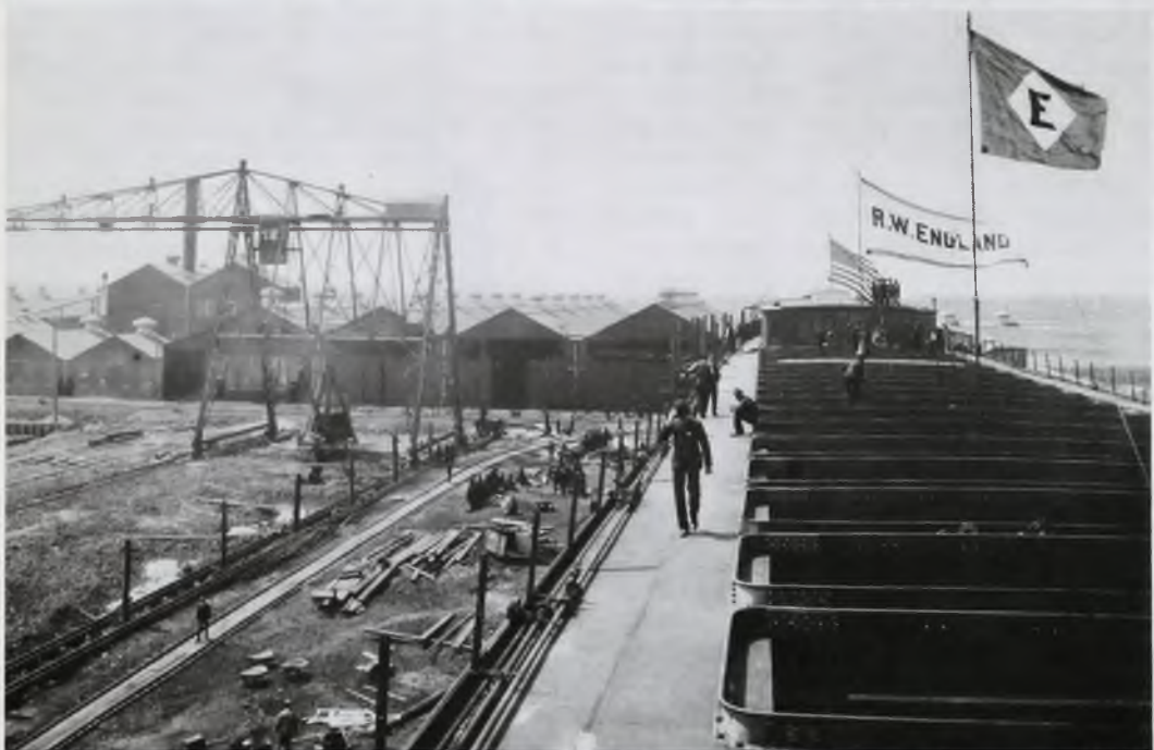
The R.W. ENGLAND was the first vessel built at GLEW and she measured 377' x 50' x 28'3".
