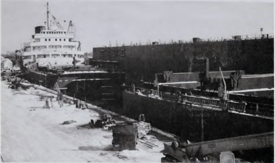
WHEAT KING lengthened at Port Weller Drydock.
