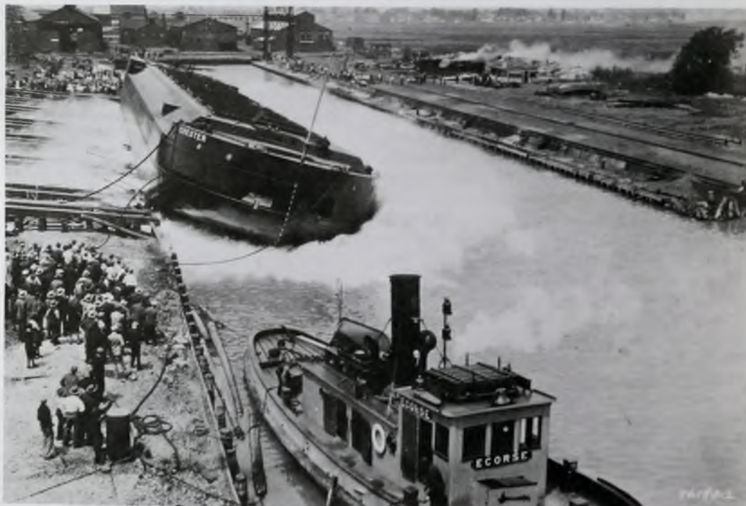
The GLEW shipyard tug ECORSE stands by to assist the CHESTER after she was launched.
