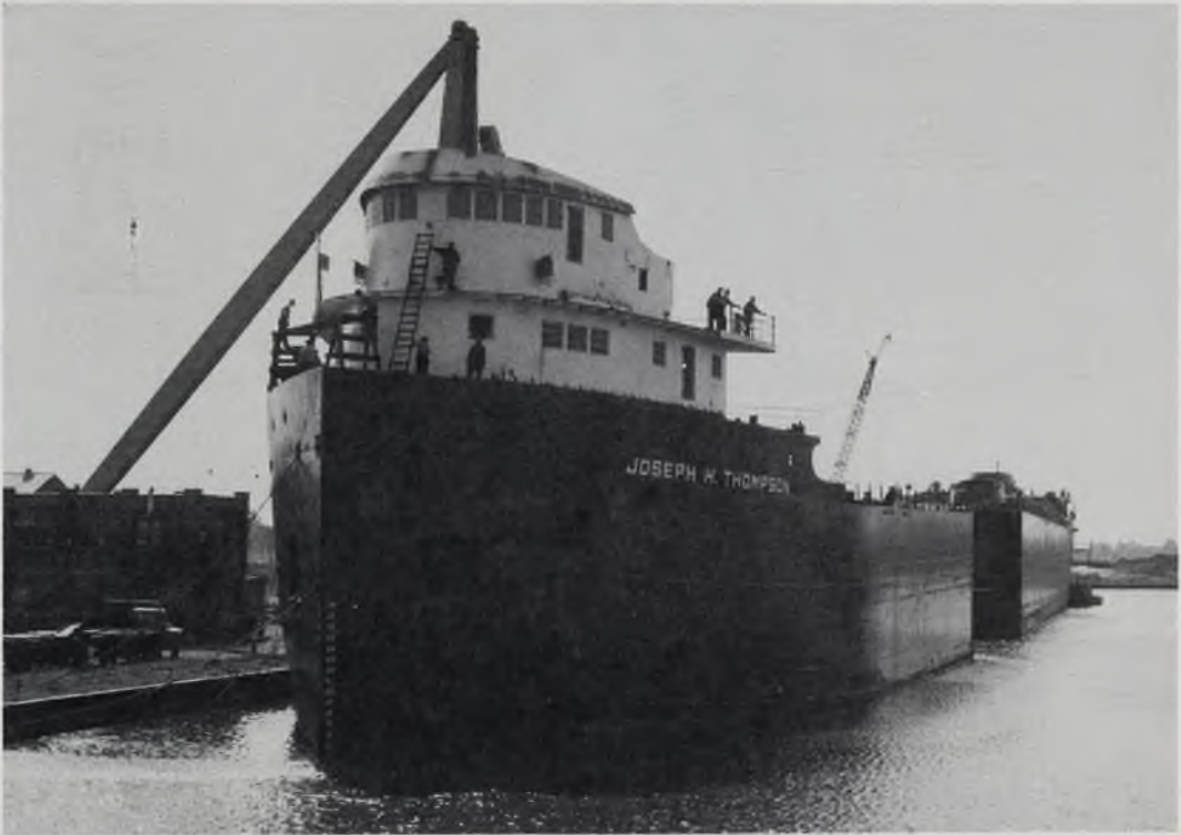
Top: The stern section with false bow and superstructures on deck arrive at Amship's yard in Chicago. Both sections are aligned together and the forward cabins attached.
