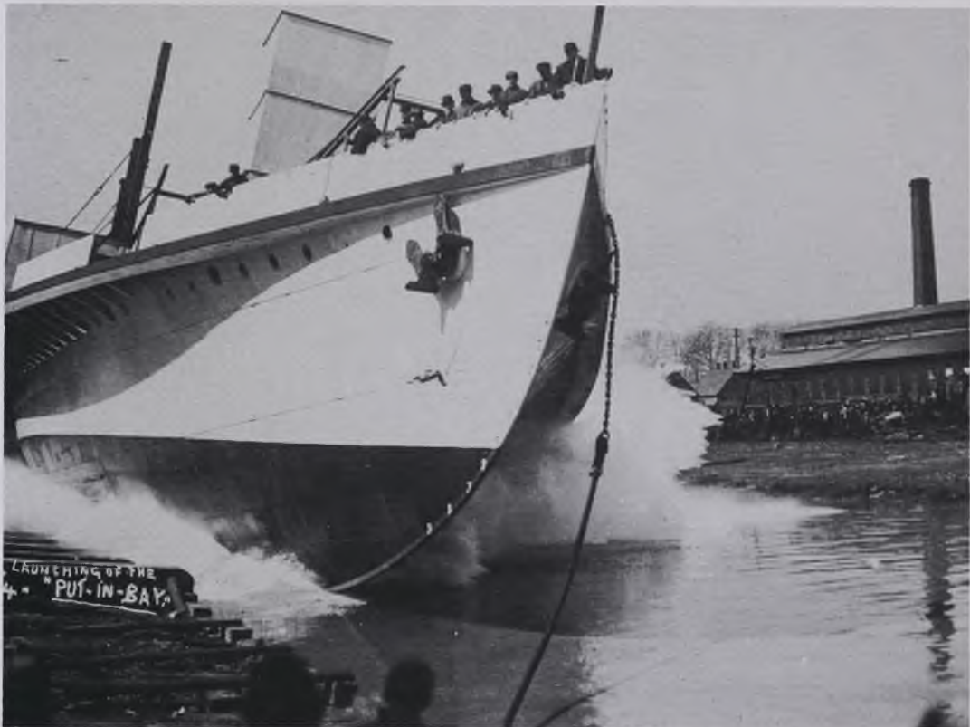
The side-launching of the PUT-IN-BAY at Detroit Shipbuilding's yard in Wyandotte, Michigan.
