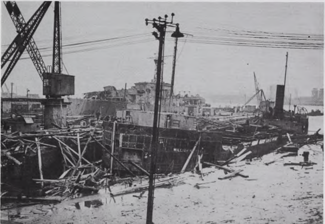
The WILLIAM H. DANIELS damaged at drydock in 1949.
