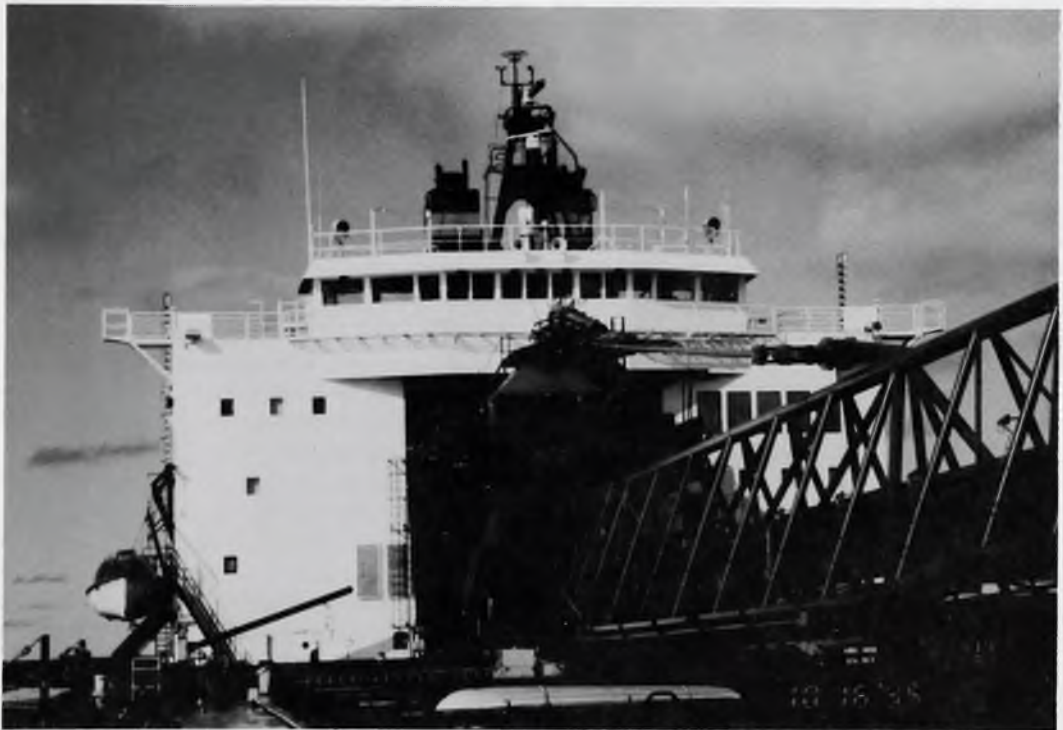
Top: The TREGURTHA was built with five cargo holds, capable of carrying 68,000 tons. Bottom: The TREGURTHA is capable of offloading 8,500 tons per hour on her 260-foot unloading boom.
