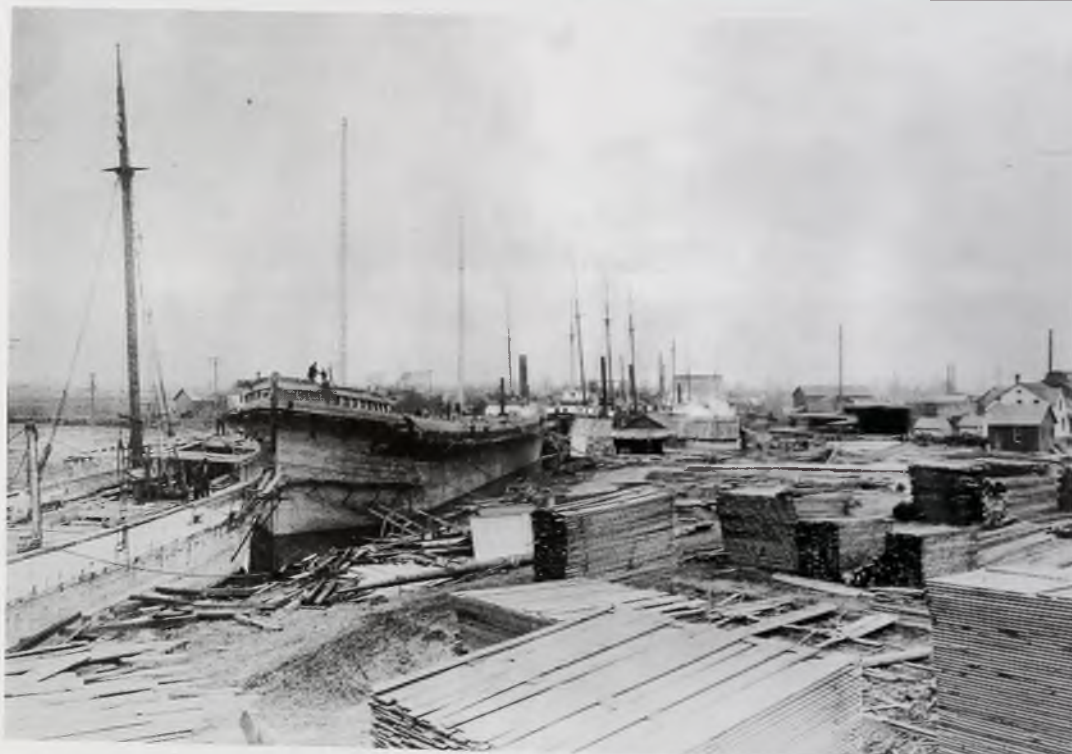
Vessels being repaired at Kenyon's Shipyard at Marine City, Michigan.
