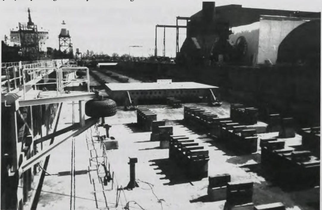
The keel for Hull #79 at Pt. Weller Dry Docks – April 1, 2000
