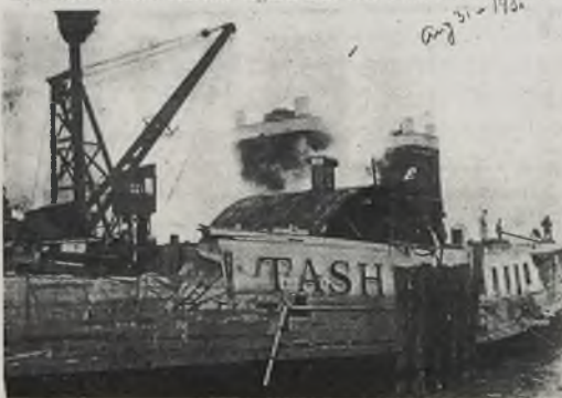
Tashmoo Makes Harbor Again But Not Under Own Power
