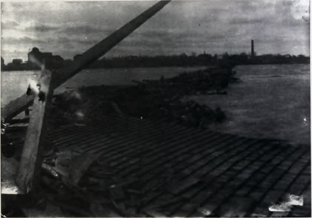
Damage caused by the storm on the docks at Pt. Hope in Michigan's Thumb. They were never rebuilt, but the remains can be seen to this day.
