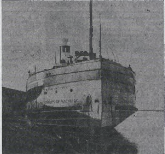
THE State ferry boat, Straits of Mackinac, as it appears with a new deck, built to carry motorists' automobiles.
