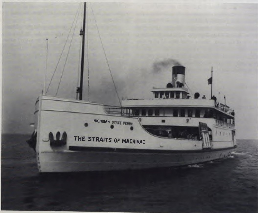
STRAITS OF MACKINAC - Built in 1928 at Great Lakes Engineering Works in Ecorse, MI Measured 190 ft. long, 48 ft. wide, 16.6 ft. depth
