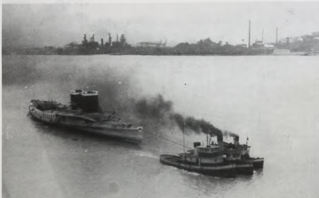
TASHMOO hull was launched on December 31, 1899 and towed from the Detroit Shipbuilding Company in Wyandotte to the Orleans Street yard for joiner work.
