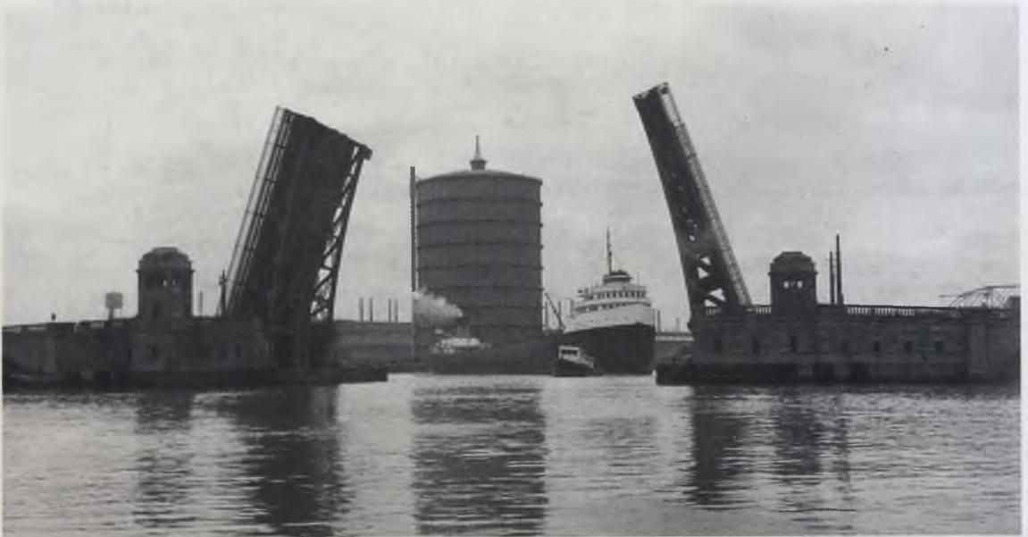
Before Bow Thrusters were installed in early 1960s, ships needed tug assistance to turn around at Ford Dock before passing thru Dix Street Bridge. Photo from Dossin Museum Collection
