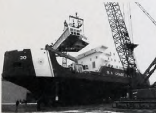
Final Assembly of the USCG MACKINAW
