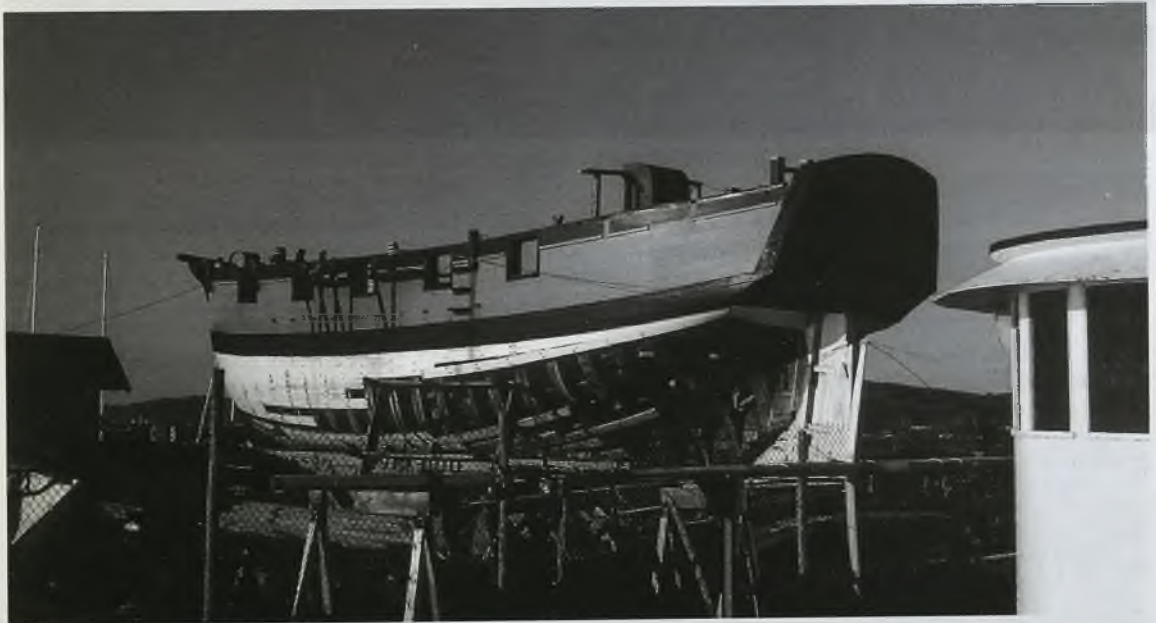
HMAS WELCOME being rebuilt at Traverse City - June, 2005
