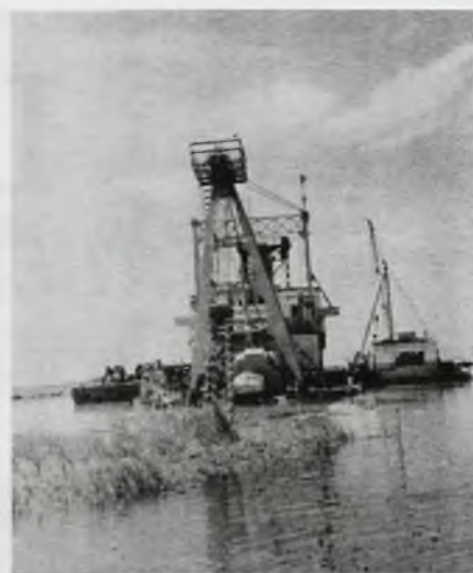
The "Business End" of the 27-inch Hydraulic Dredge CARTEGENA boring into the depths of the St. Clair River at Southeast Bend. The total amount of material removed, 22,000,000 cubic yards of sand and soft clay would cover the entire area of Belle Isle for a depth of 15 feet.
