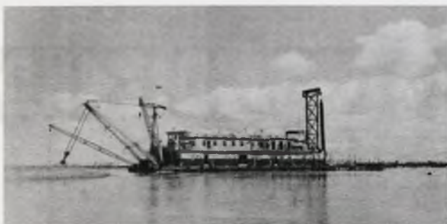
A big cut-up on the lower St. Clair River is the hydraulic dredge SHUNIAH engaged in scooping out the new Southeast Cut-off channel. It is part of the multi-million dollar Great Lakes connecting channels project started by the United States Army Engineers in 1957.
