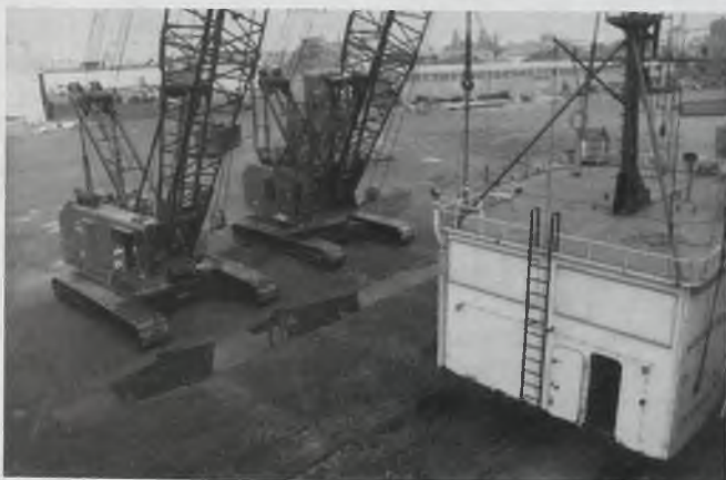
Pilothouse stored at Detroit Marine Terminal
