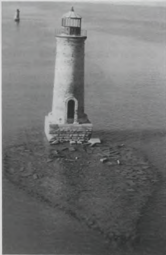
View of Rear and Front Range Lights, 1988.
