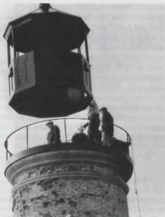
The restored Rear Light Lantern Room was installed October 13, 2005.
